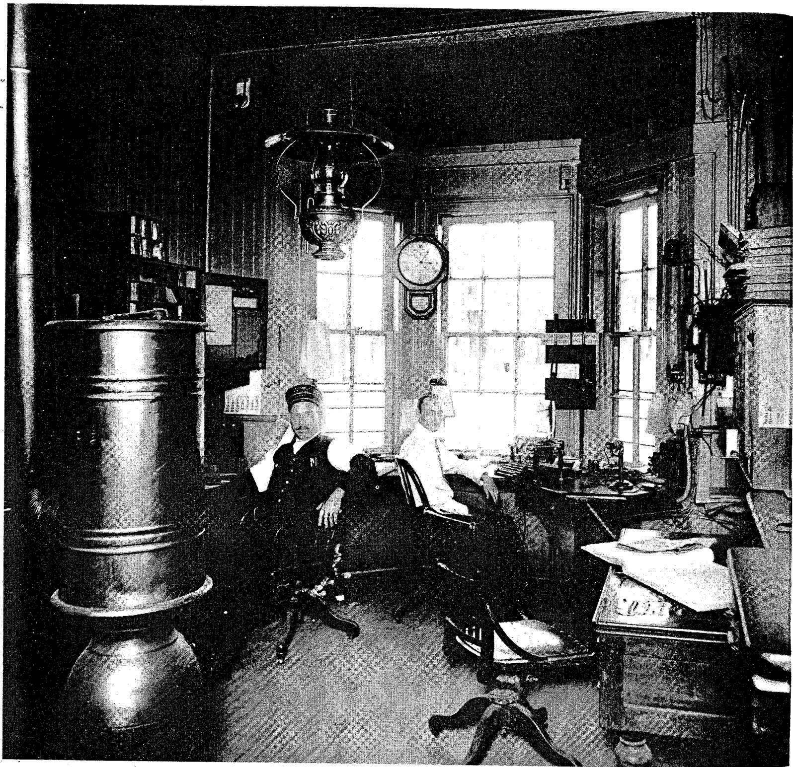
Inside the little red depot, which was moved here on a flat car from Deer Grove in 1854. It was later enlarged, then moved to the west side of North Hough Street and used as a freight depot. Photograph in 1914.
