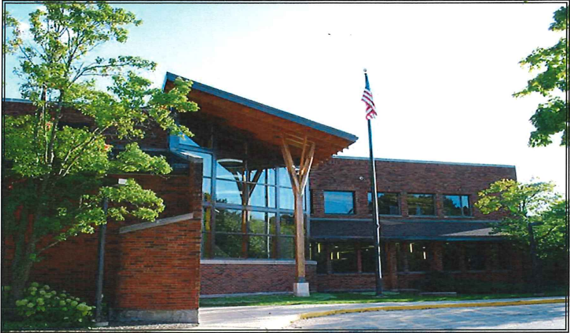
WEST END OF NORTH ELEVATION OF LIBRARY
