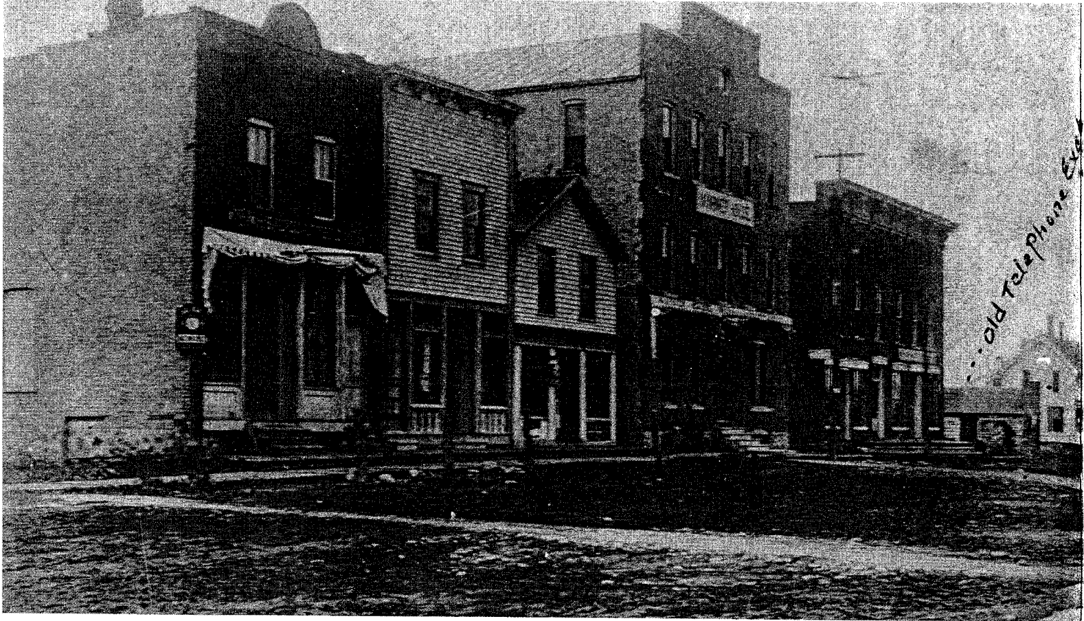
East Main Street block after it was rebuilt after 1890 fire. These buildings were on north side of East Main just east of railroad tracks.
