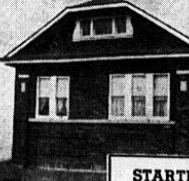
The Wernickes home at 15741 Marshfield Avenue, Harvey, Ill. Over 20,000 Chicago-land homes have installed gas heat.
